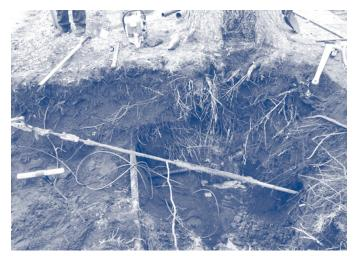
Service Line Replacement with K Copper Using cable and backhoe to complete work related to Michigan's new Lead and Copper Rule
