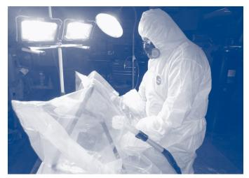
Asbestos Gasket Removal from Diesel Generator Staff wear personal protective equipment when handling materials that may contain asbestos
